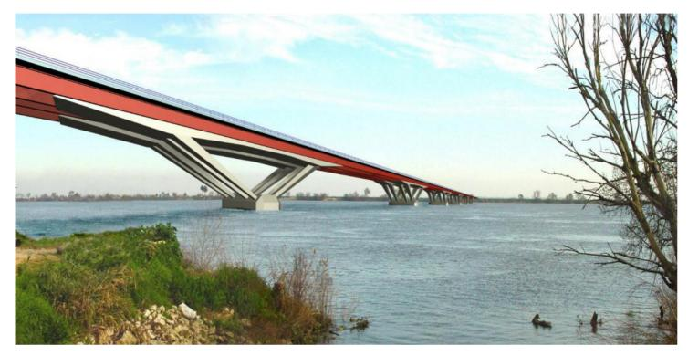
The proposal presented for the new bridge over the River Tagus in Carregado is divided into three structures; the main bridge over the river and the north and south approach viaducts. The total length reaches 11,545.0m divided into 1,442.5m for the North Viaduct, 965.5m for the main bridge and 9,141.0m for the South Viaduct.
